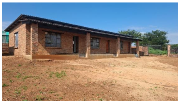
Figure 1 Three classrooms that will be used for the creche
